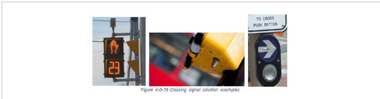
Figure 87: Crossing signal solution examples (Source: Consultant, 2015)
