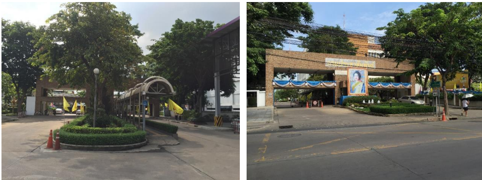
Figure 3A-4-131 Location D: The Government Public Relations Department gate (Source: Consultant)
